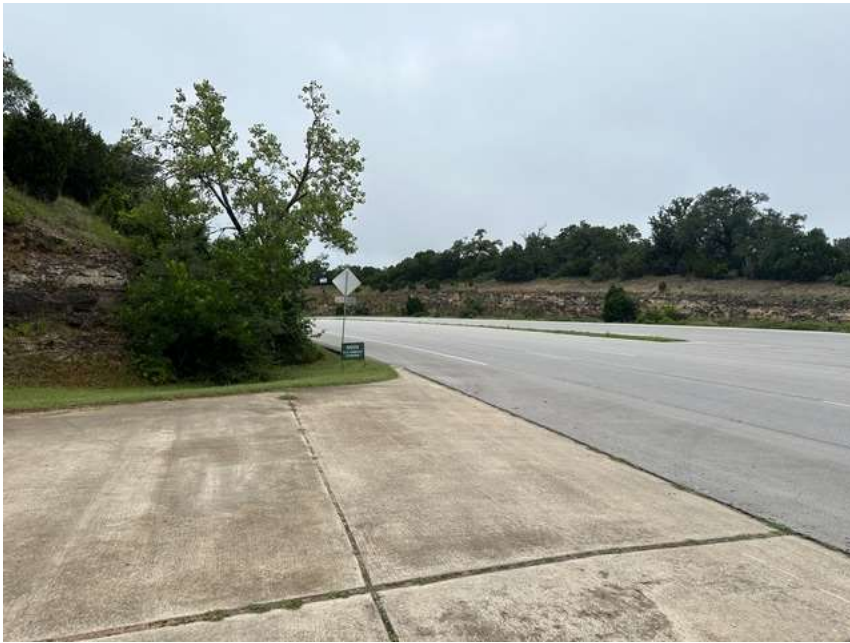
Dangerous “Blind” Ingress and Egress
